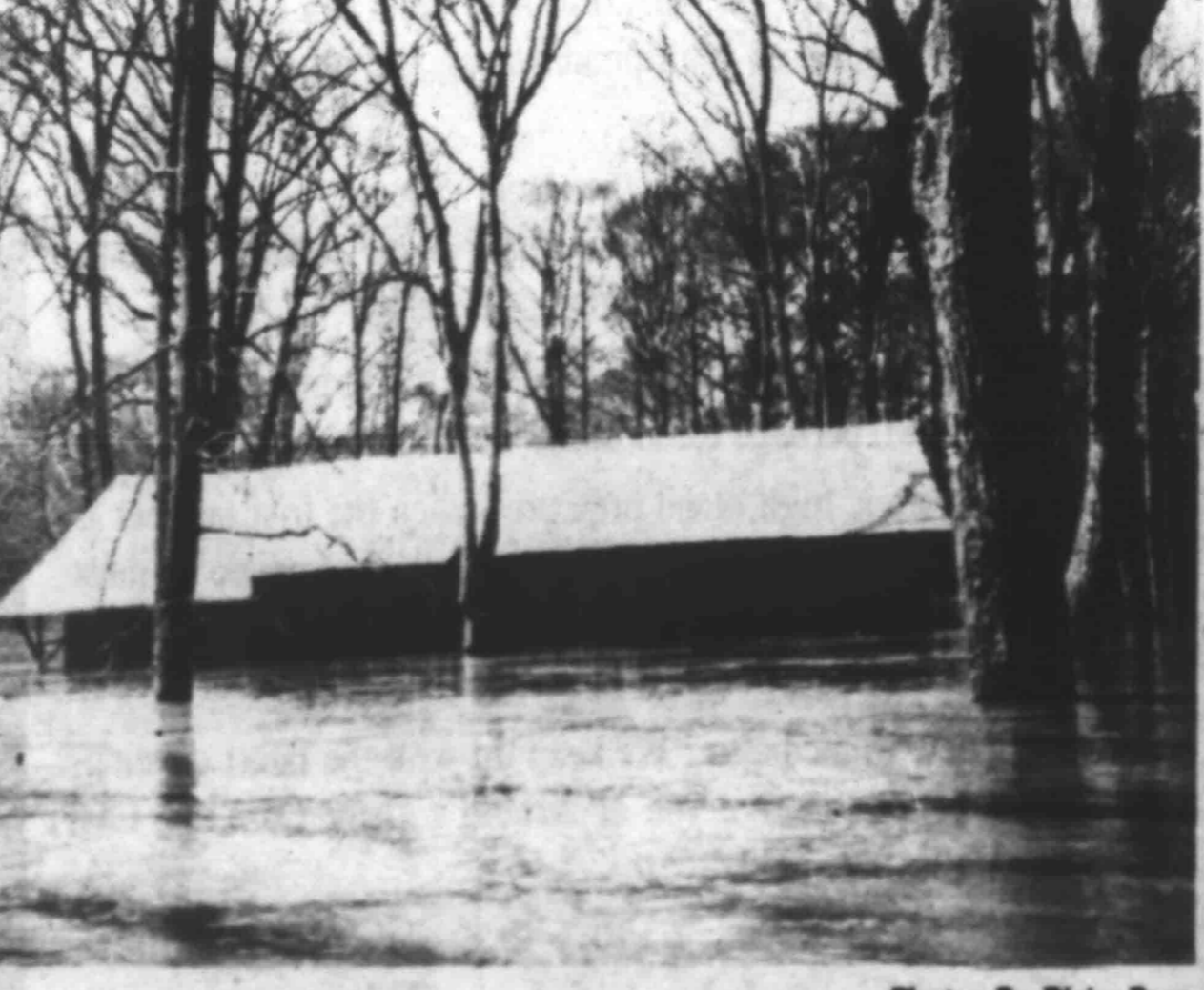
WATER FLOODS HOUSE on Open Lake.
